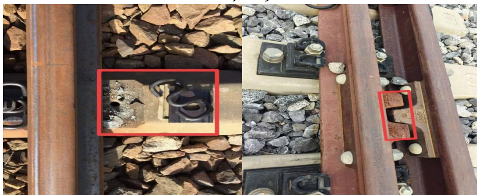
Figure 6: Close-range track equipment detection (fasteners, sleepers)
